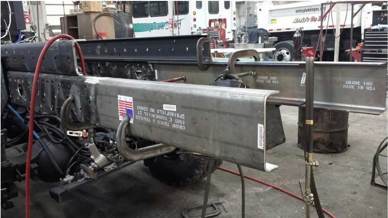
Welding the lower frame rail extensions on.
